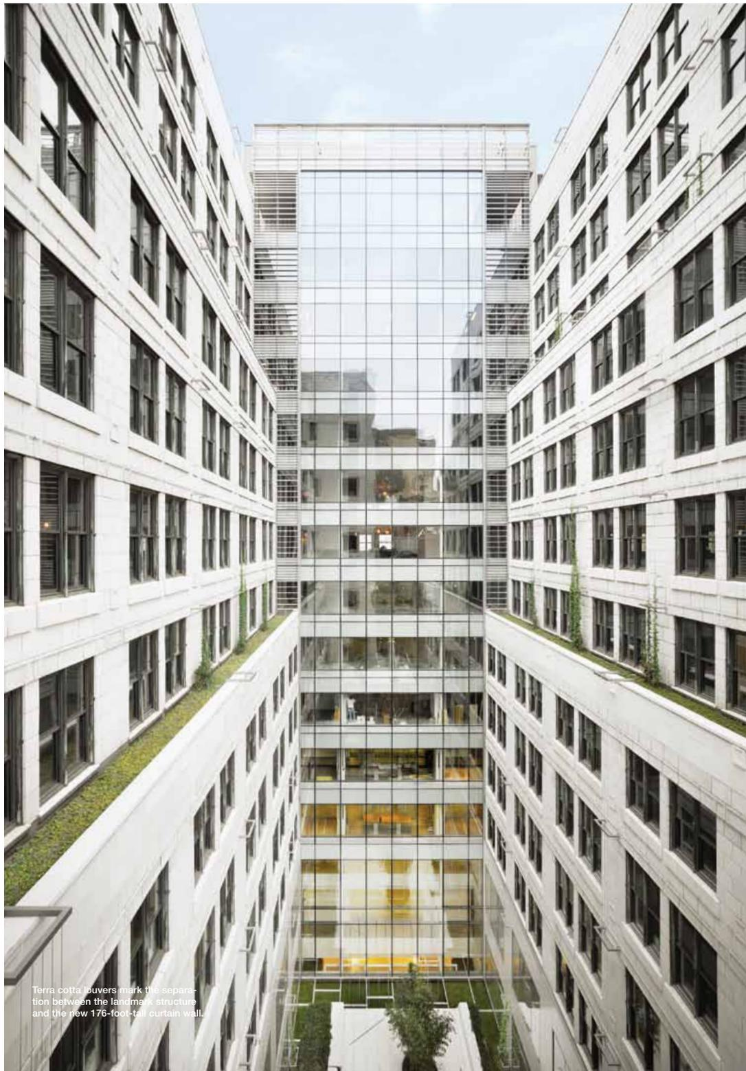
Terra cotta louvers mark the separation between the landmark structure and the new 176-foot-tall curtain wall.
