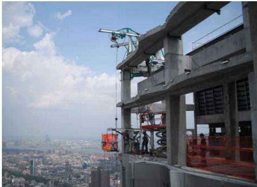
**Above** Curtain wall erectors install 9-foot-10-inch-tall curtain wall sections ranging in width from 3½ to 5½ feet high above lower Manhattan.
