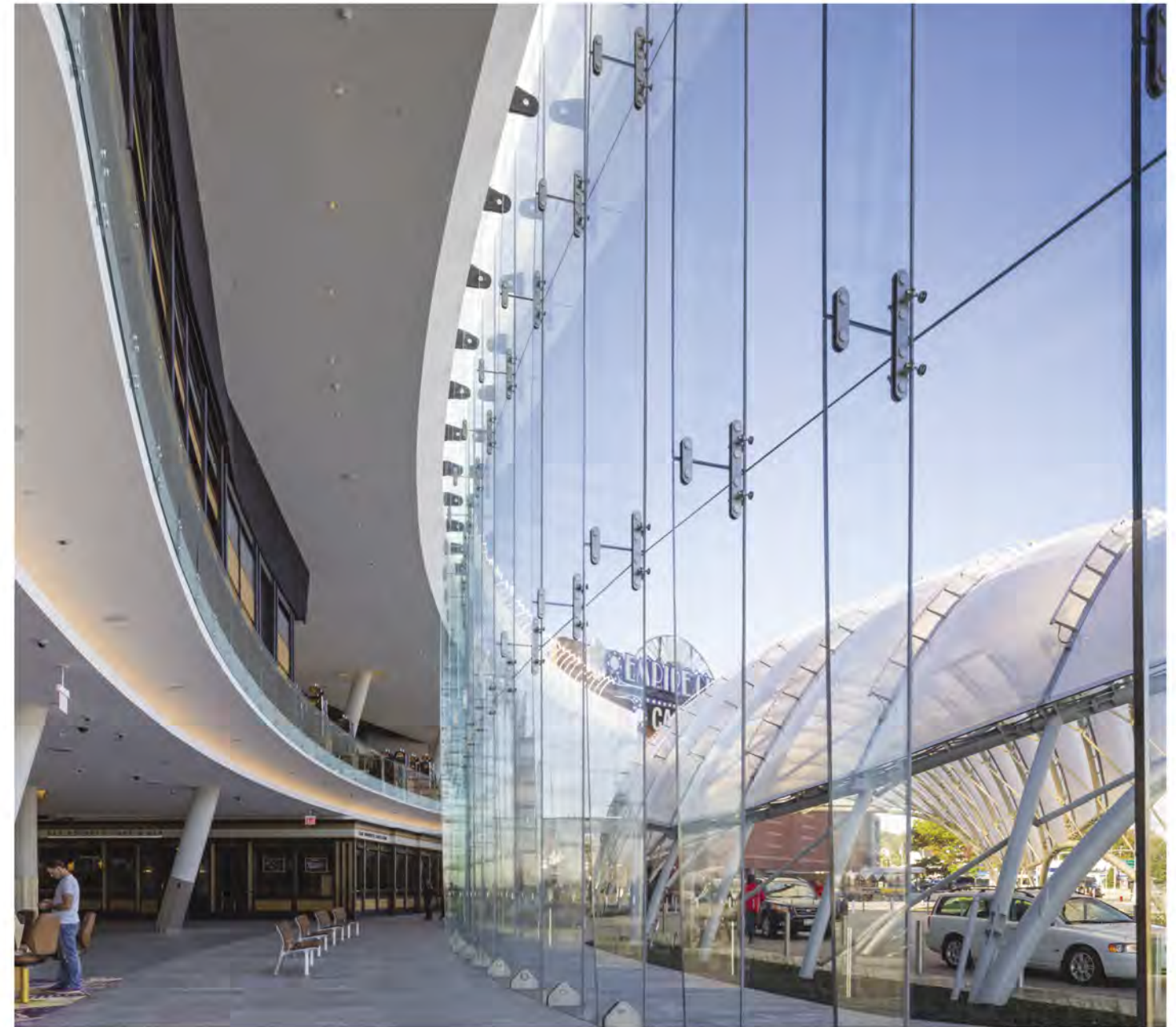
Above A four-story facade of frameless, low-iron glass forms the 300-foot arching facade of the new casino.
