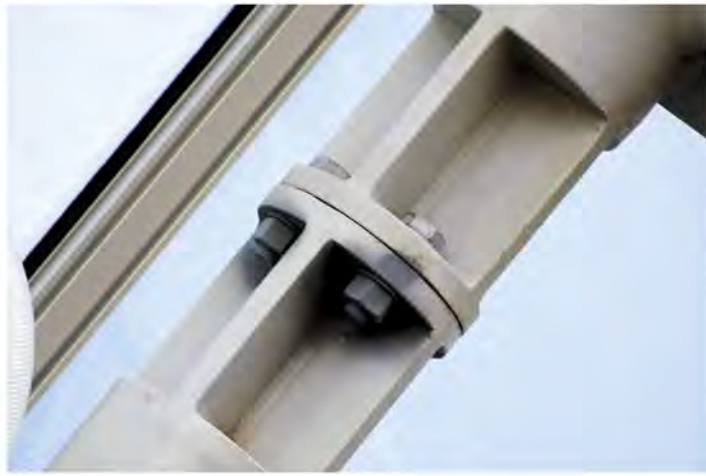
Above A system of 8-inch-diameter steel arches and 4-inch-diameter purlins created efficient geometric connections, reducing construction costs.
