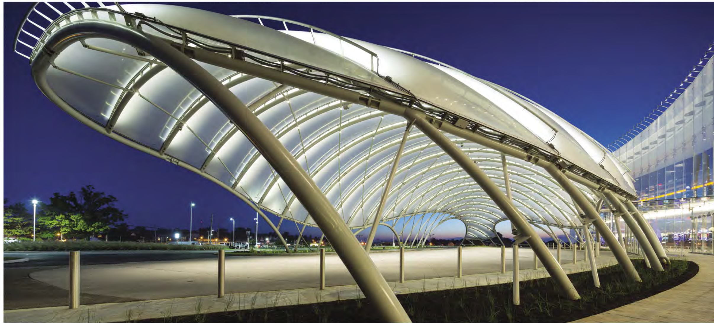
This spread The lattice-shell porte-cochère and 45-foot-tall glass curtain wall create a dramatic visual identity for the new casino.
