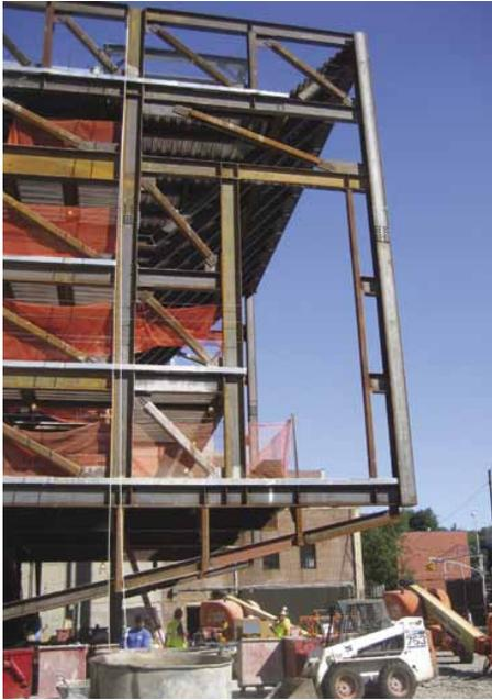
**Above left** Construction photos reveal the structural steel beams that support the Polonsky's cantilevered front curtain wall, with ample diagonal members. **Above right, top and bottom** The tight site in the Downtown Brooklyn Cultural District posed challenges during construction of the hybrid structural system, a steel frame in front and CMU in back.
