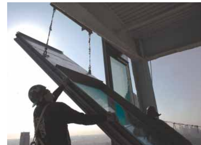
Facing and above The wall is a stacking system of unitized panels that slide into the panel below and clip in above.
