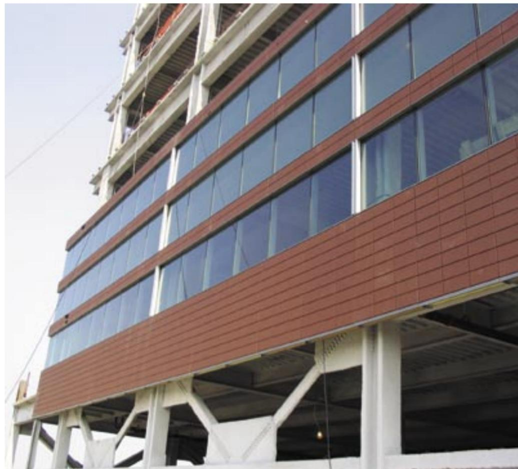
**TOP, OPPOSITE** The unitized curtain wall system allows for easy erection and replacement.
