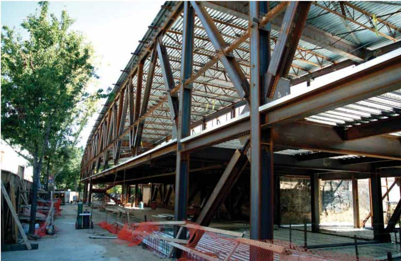
**Above** A truss on the second floor creates long column-less spans for unbroken windows along the facade.
