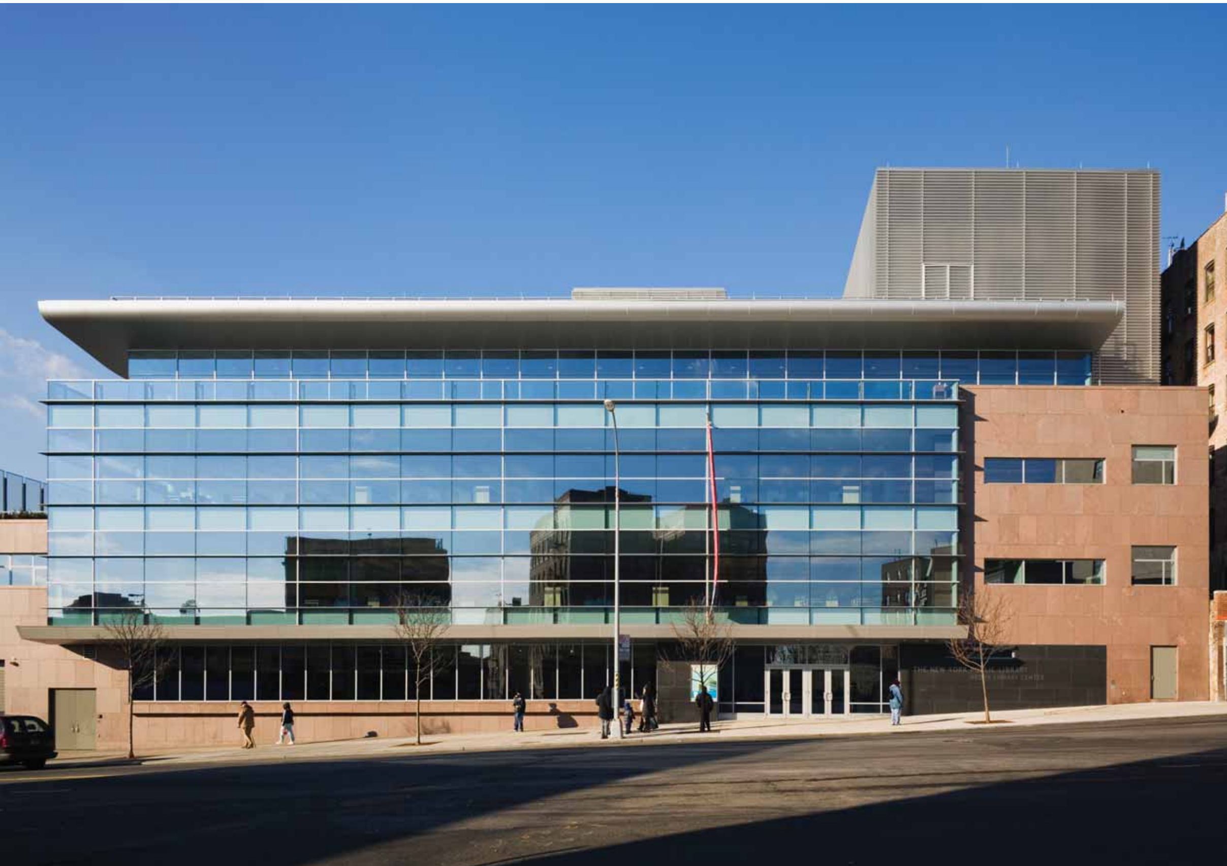
ABOVE The curtain wall's low-e glass carefully modulates daylight within the library.
