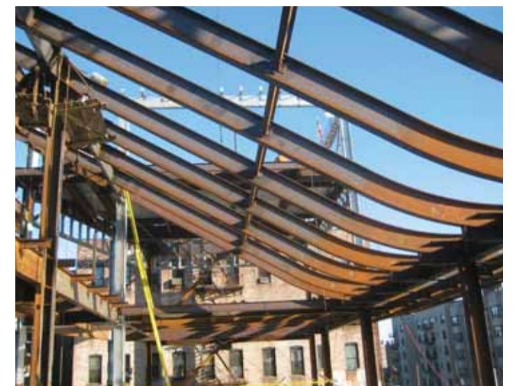
TOP The structure's primary load bearing columns await erection.
