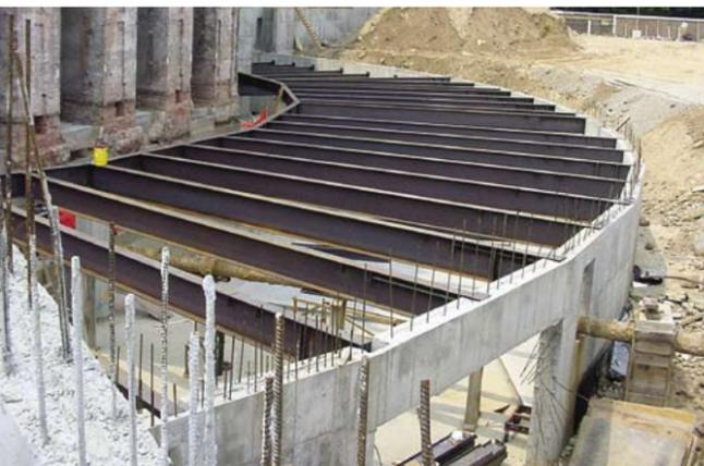
**TOP, ABOVE LEFT** Steel floor framing above a new basement level supports the pavilion concourse.
