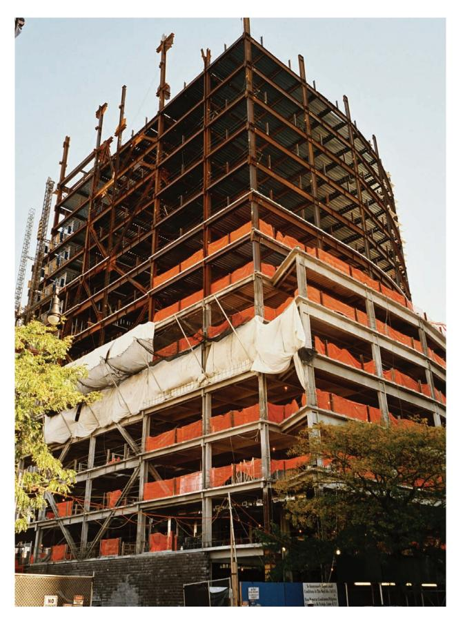
**PREVIOUS** LIC 2's elegantly placid facade hides a complex structure designed to handle the anticipated loads of a significant addition.
