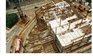
ABOVE With the exception of the welded perimeter moment frames, all of the connections were bolted
