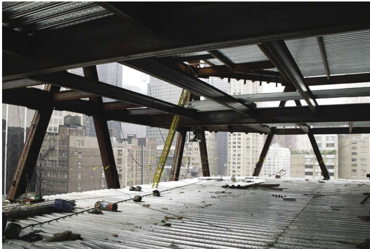
TOP Ironworkers connect the initial bolts of a 6-ton node connector
