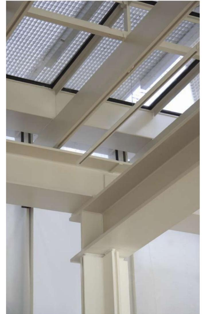
that are welded to the sides of the flanges. The cube is braced with 9-by-5-by-5/8-inch tubes, and its A36 plate steel cladding is coated with white intumescent fireproofing paint and finish coated with an off-white architectural paint to echo the stone facades of the existing buildings.
