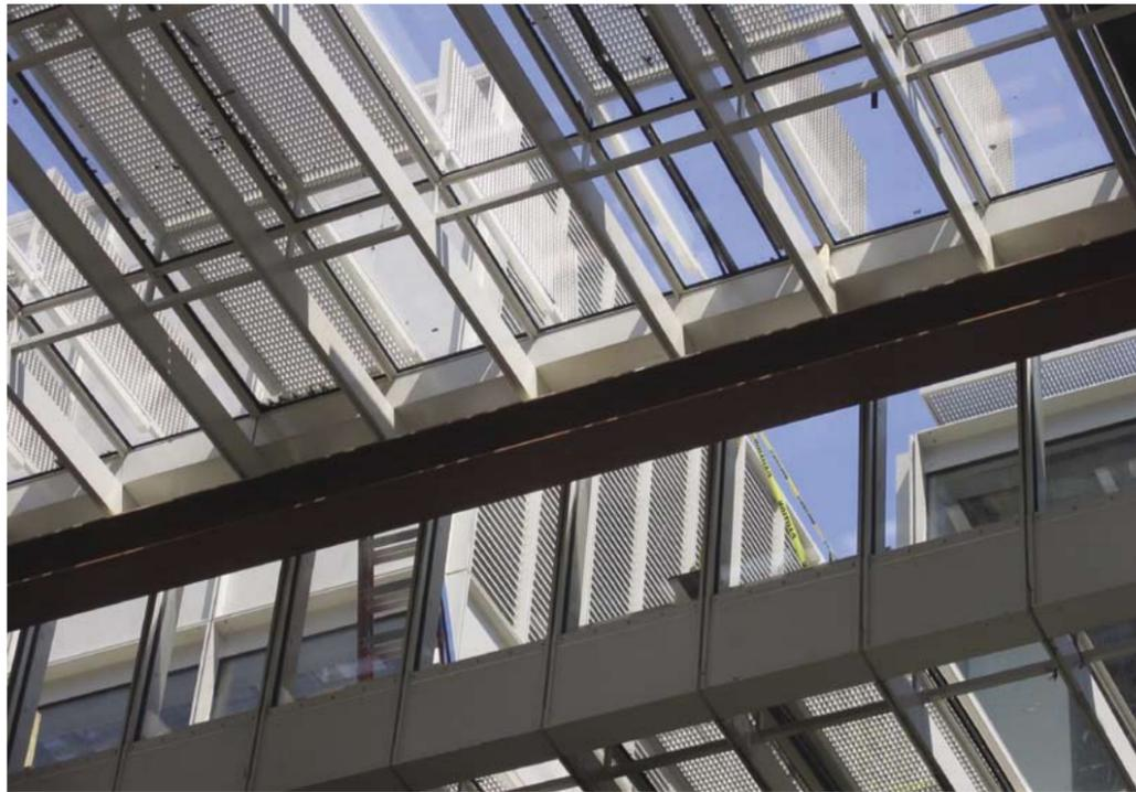
**RIGHT** Moment connections bond the cruciform columns to the girder beams, while the skylight is attached to this structure by way of adjustable clips.
