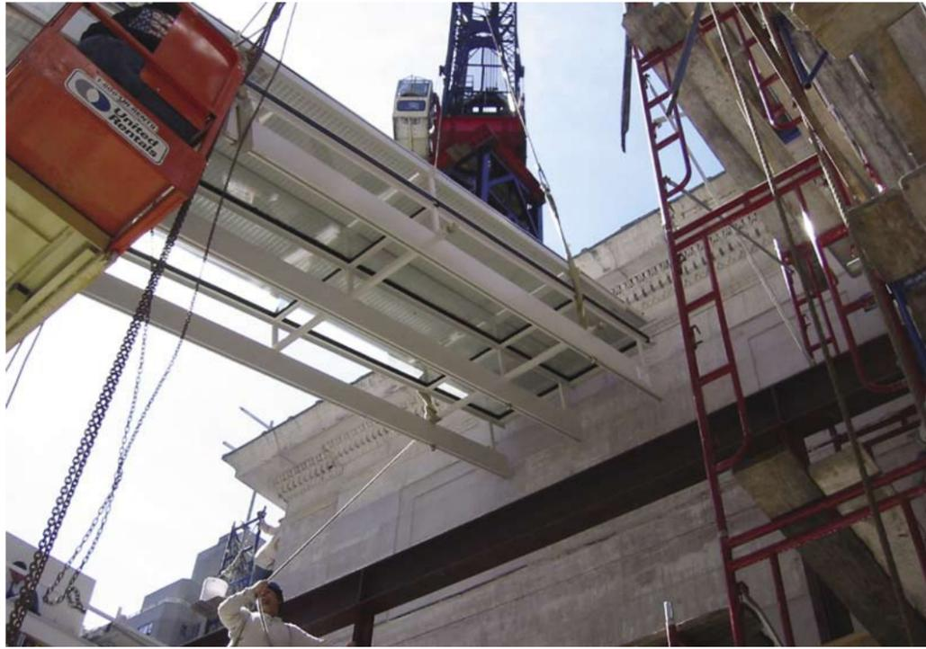
**TOP** A 6-foot-wide-by-30-foot-long section of skylight, prefabricated in Germany, is lowered onto supporting steel girders.
