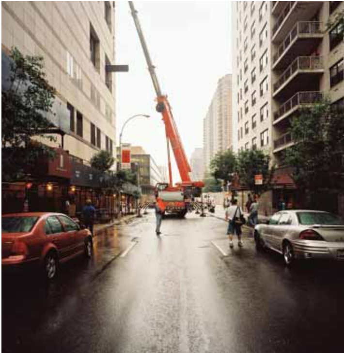
Clockwise from top left The 44-foot long, W36x328 beams were delivered on site by truck, then crane lifted and inserted through a window in the building.
