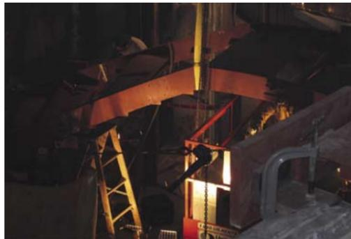
**ALL ABOVE** The stair was shop fabricated in eight pieces, then welded on site in two segments.
