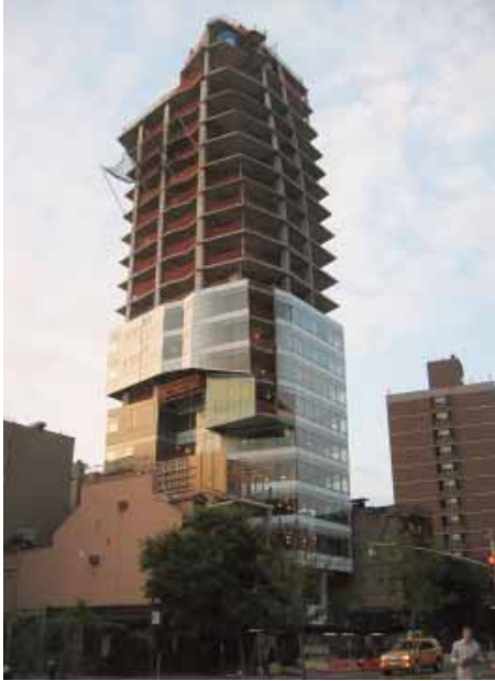
Above Curtain wall panels were manufactured in the Josef Gartner factory before being mounted into concrete-slab anchor channels.
