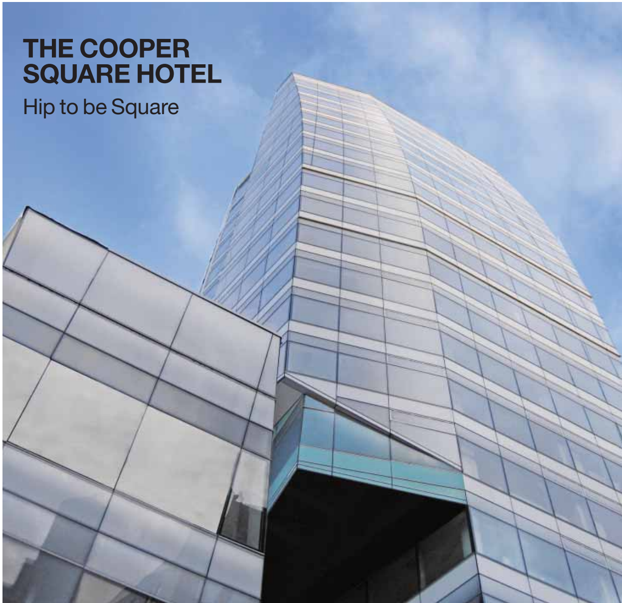
Left The glass, aluminum, and ceramic curtain wall designed by Carlos Zapata Studio accentuates the building's height with shifts of material and pattern.
