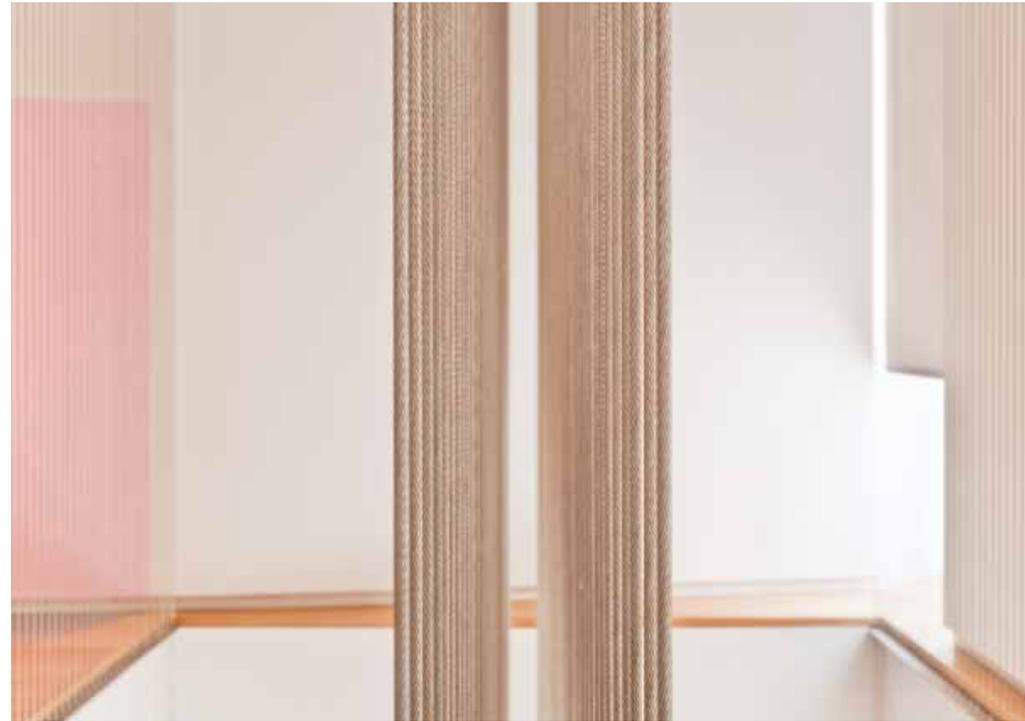
**Facing above** Cables were tensioned by hand at the structural supports, then manually threaded through their corresponding holes and clamped and pinned to the stair's treads.
