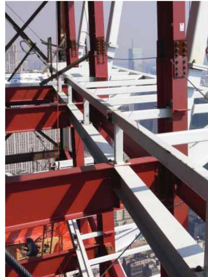
Above The screen wall framing cantilevers up from the roof and is topped by a stiffening truss.
