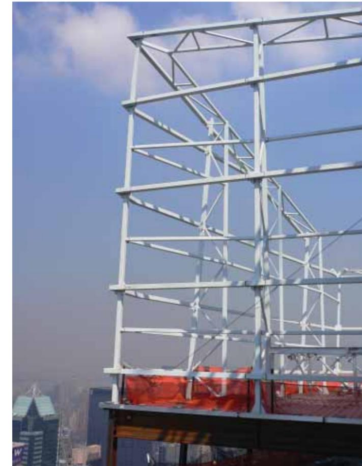
kept as thin as possible around the perimeter of the building to maximize rooftop area for mechanical equipment. It also makes way for One Bryant Park's nearly 300-foot-tall spire. Built mainly of large-diameter, shop-welded steel pipe, the spire tapers from 5-foot-10-inch-diameter at its base to 2-foot-2-inch-diameter at the tip, where it makes the tower New York's second tallest after the Empire State Building.
