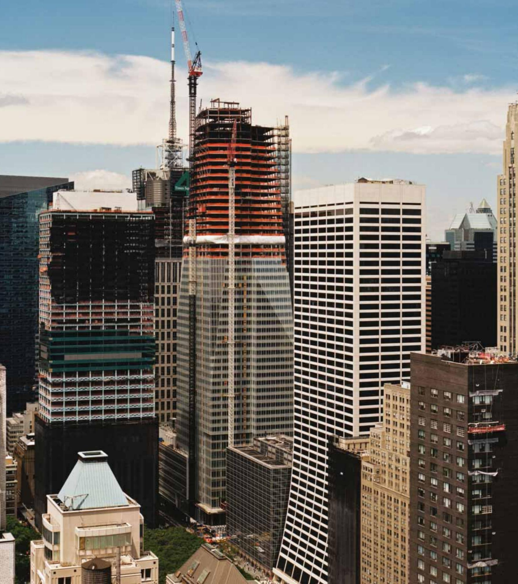
**Facing** Steel framing allowed generous 14-foot-6-inch floor-to-ceiling heights while maintaining slim column profiles.
