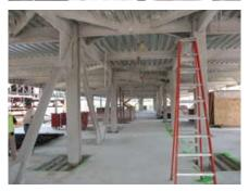
Above Thirty-foot spans allow for the placement of one classroom per bay. Columns are connected to the slab with %-inch diameter studs, allowing doors, lockers, and large windows to be placed in between.
