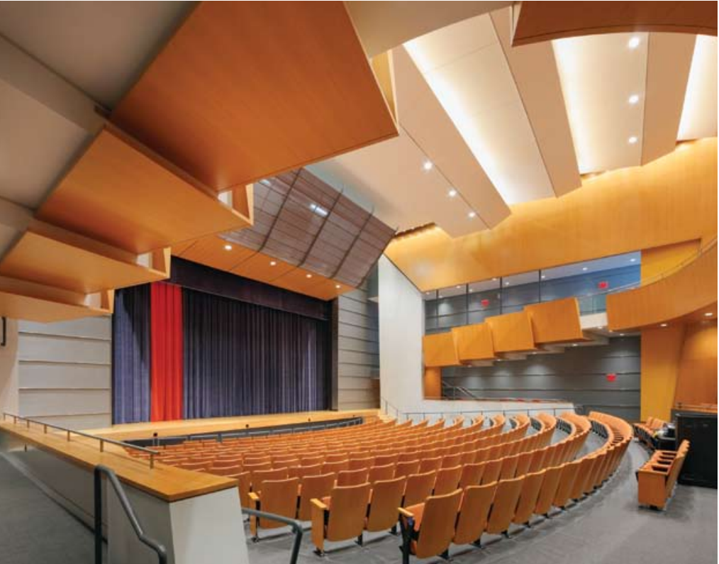
Above The theater incorporates a fly loft and a raked and cantilevered balcony. Below Glass-enclosed studio spaces, with views to the north and east, are stacked atop a 20-foot cantilever.
