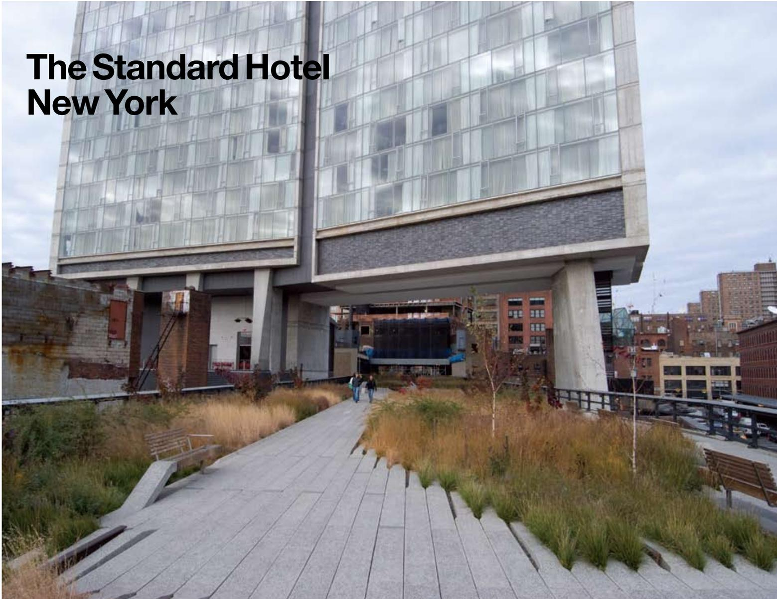
Left A steel truss anchored to the eastern concrete pier and to the Standard's western shear wall allows the hotel to make a 100-foot straddle over the High Line.
