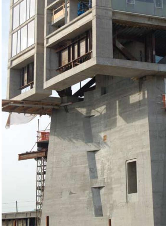
the 24-month construction cycle. A single tower crane with an adjustable 150-foot boom erected on the northern edge of the eastern concrete pylon was used to hoist the truss members onto a series of three shoring towers and a cantilever support. Once the trusses were joined in the center and secured to the shear wall and pylon, the contractors were able to extend the boom to pick the lighter loads of the remaining material.
