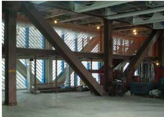
that transfer the gravity load down to bedrock.
