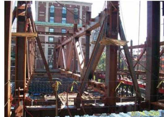
**Facing** The building was constructed using Building Information Modeling (BIM). Lab floors are framed with 5-foot-deep castellated beams to allow 18-foot floor-to-ceiling heights that make room for office mezzanine levels. A unique tower crane design with a bumped-out base made room for truss assembly atop a heavy construction shed.
