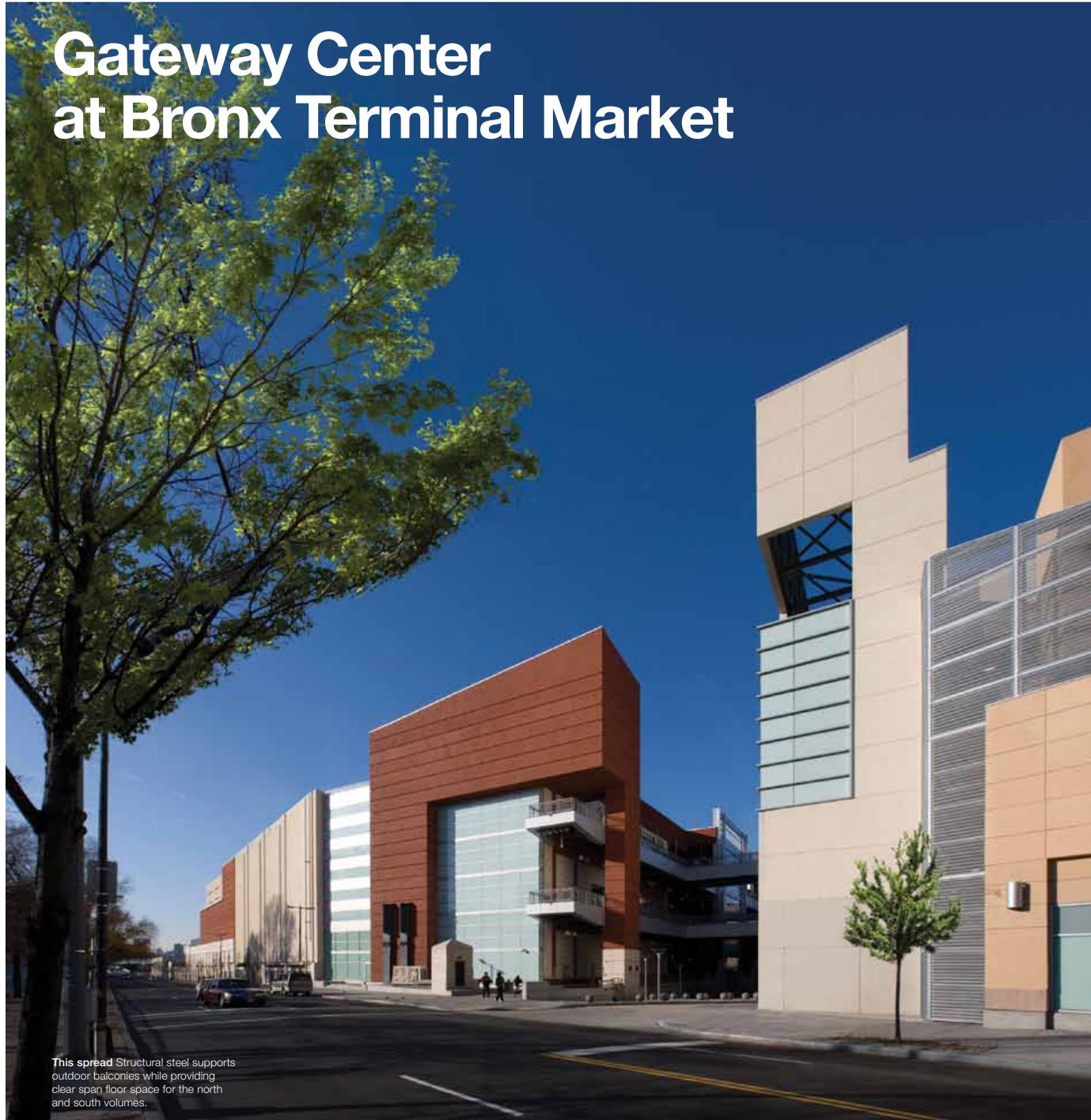
This spread Structural steel supports outdoor balconies while providing clear span floor space for the north and south volumes.
