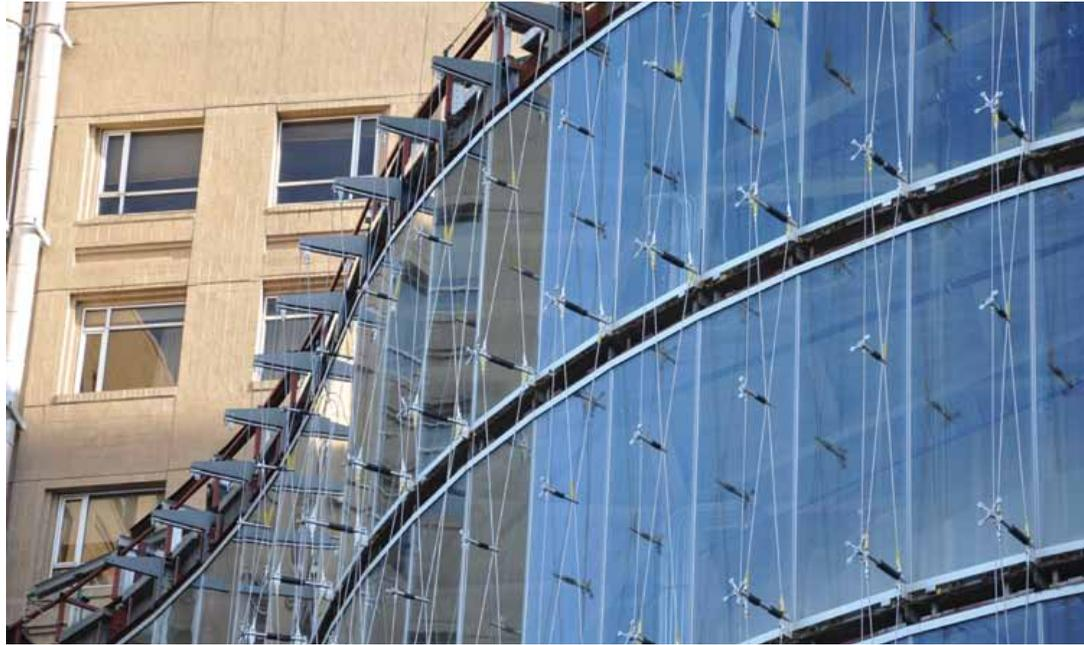
high performance glass would have a shading coefficient of .6 to .45," says Bader. "The shading coefficient of this system is very low—.1 or .05. You would have to have a virtually opaque wall to get that." In addition to the blinds, the airspace features a stainless steel catwalk system, a custom grating supported by small-diameter pipe members integrated into the climate wall support structure, that allows easy access for maintenance.
