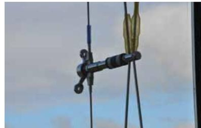
**Right** Because the climate wall structure is in tension, less material was required to handle applicable loads and steel rods could be a slender 3/8-inch diameter, making them nearly invisible from the exterior.
