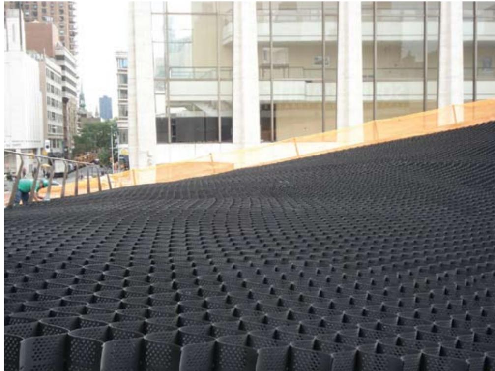
**Left** A soil confinement system, a honeycomb-like web, is stretched over the roof to stabilize the soil until roots are established.
