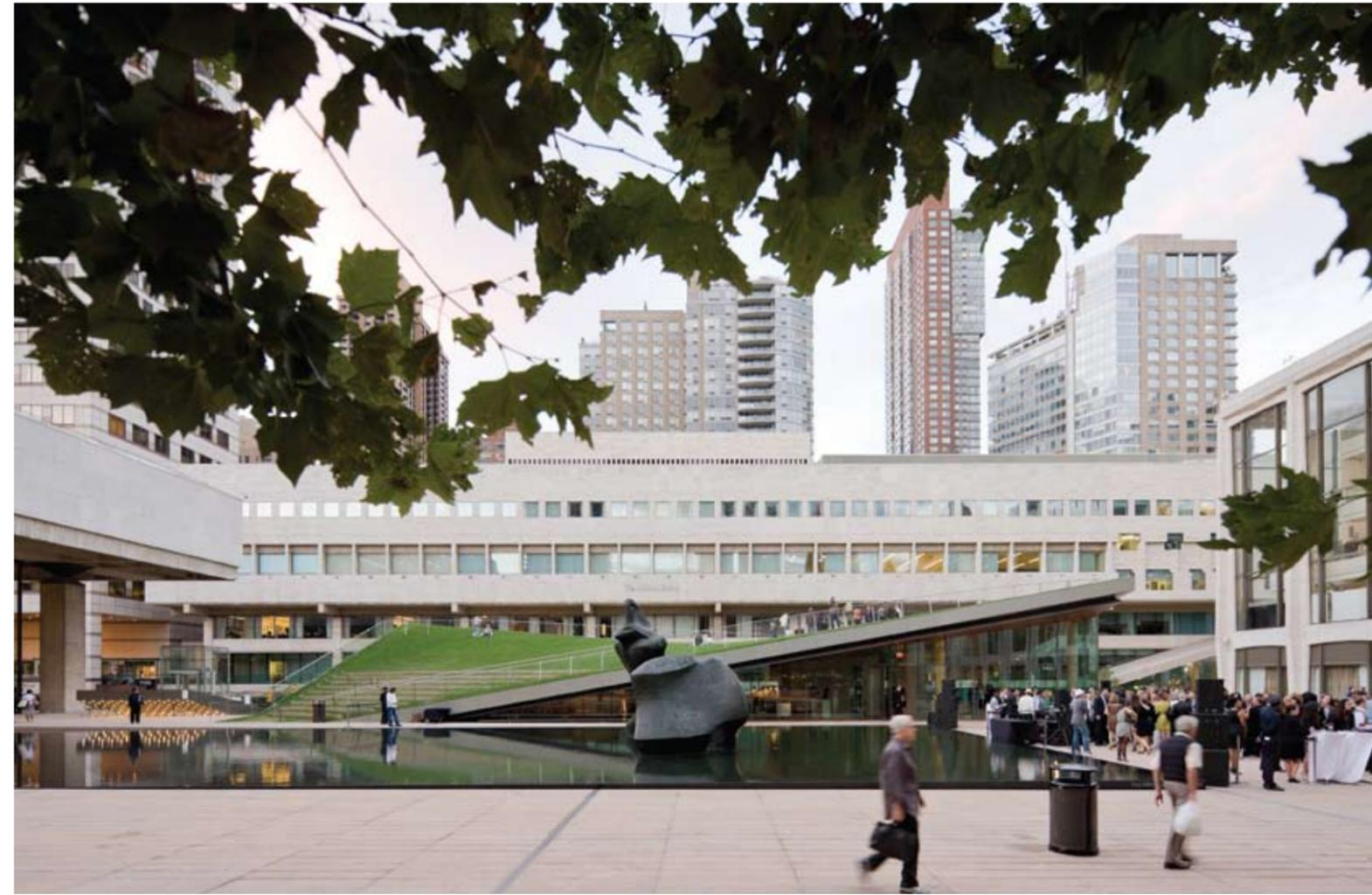
**Above** The pavilion rises next to the Paul A. Milstein Pool and Terrace. The light-weight steel structure allowed the design team to build atop Lincoln Center’s existing podium and columns.
