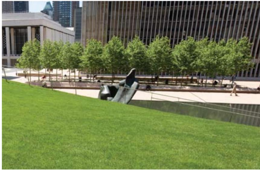
**This page** The lawn's stainless steel rail and mesh infill required precise detailing because the angle of the stanchion to the lawn surface varied between points.
