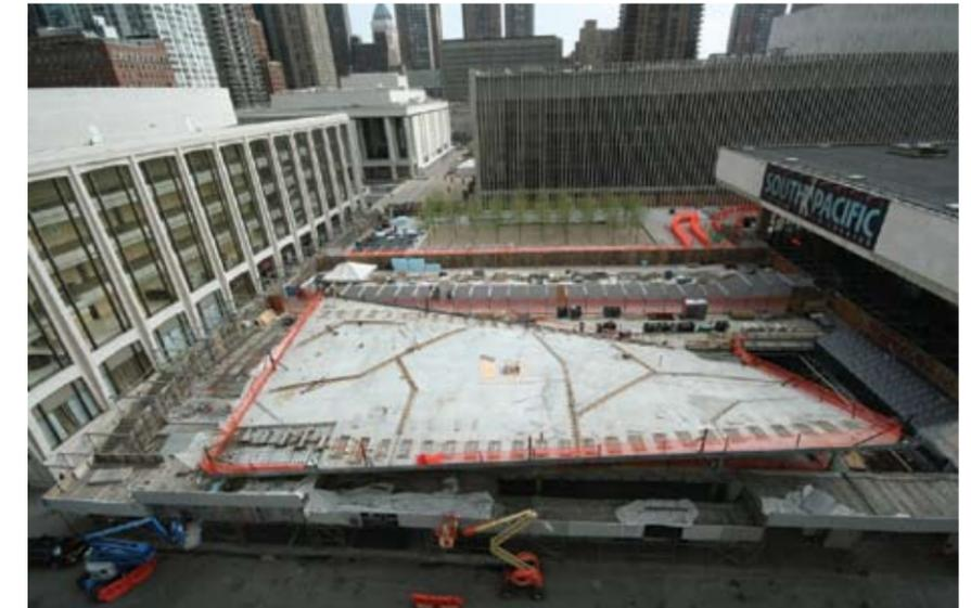
**Right** The completed steel frame is covered with a concrete deck; zigzag elements are future "check-dams" that divert storm water to strategically located drains.
