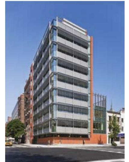
**A sheltering facade of zinc panels and aluminum louvers lets filtered daylight in while keeping autistic students focused on the lessons at hand.**
