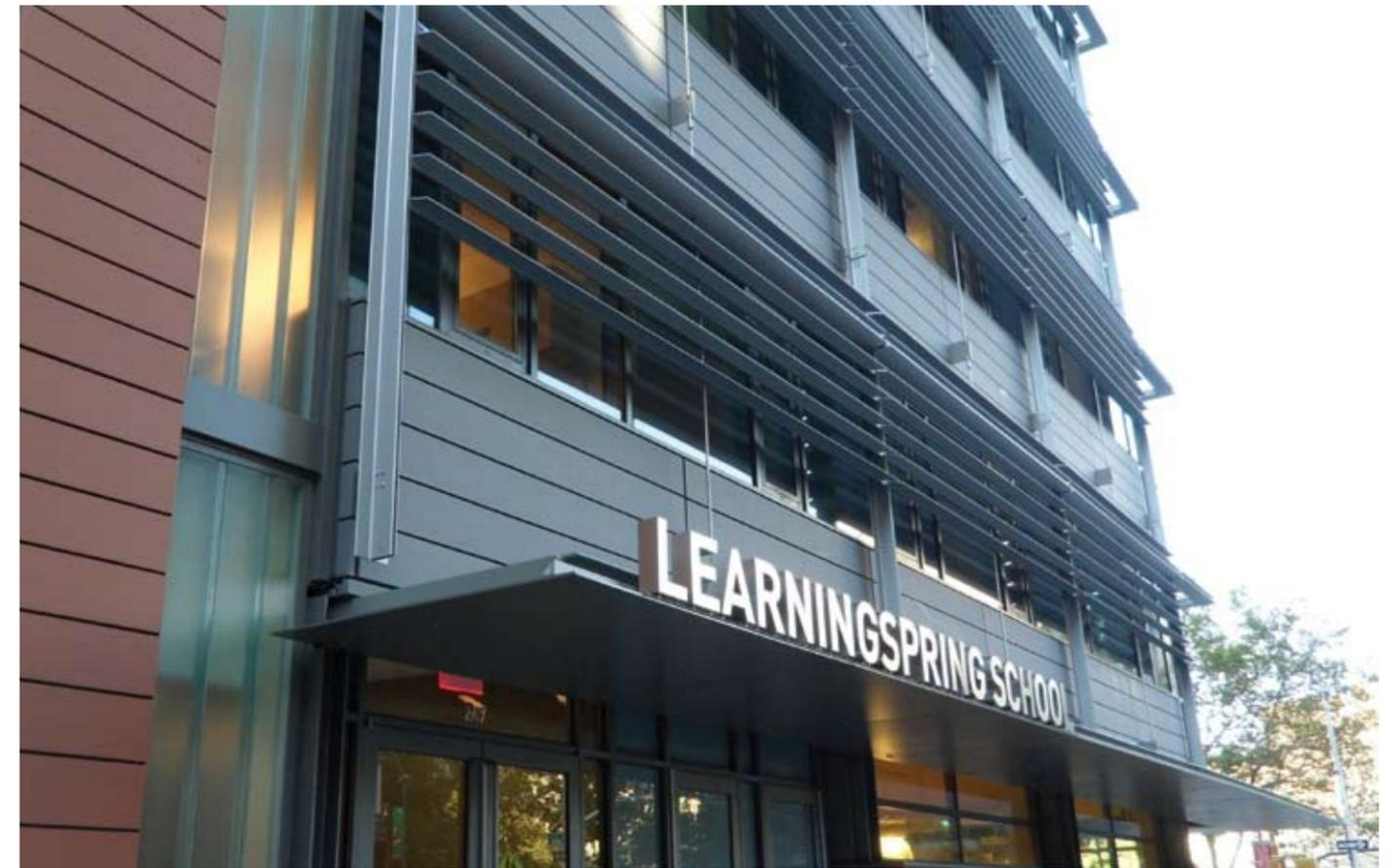
**Facing** Sunshades built from 5/16-inch-thick aluminum plates span 18- to 20-foot column bays.
