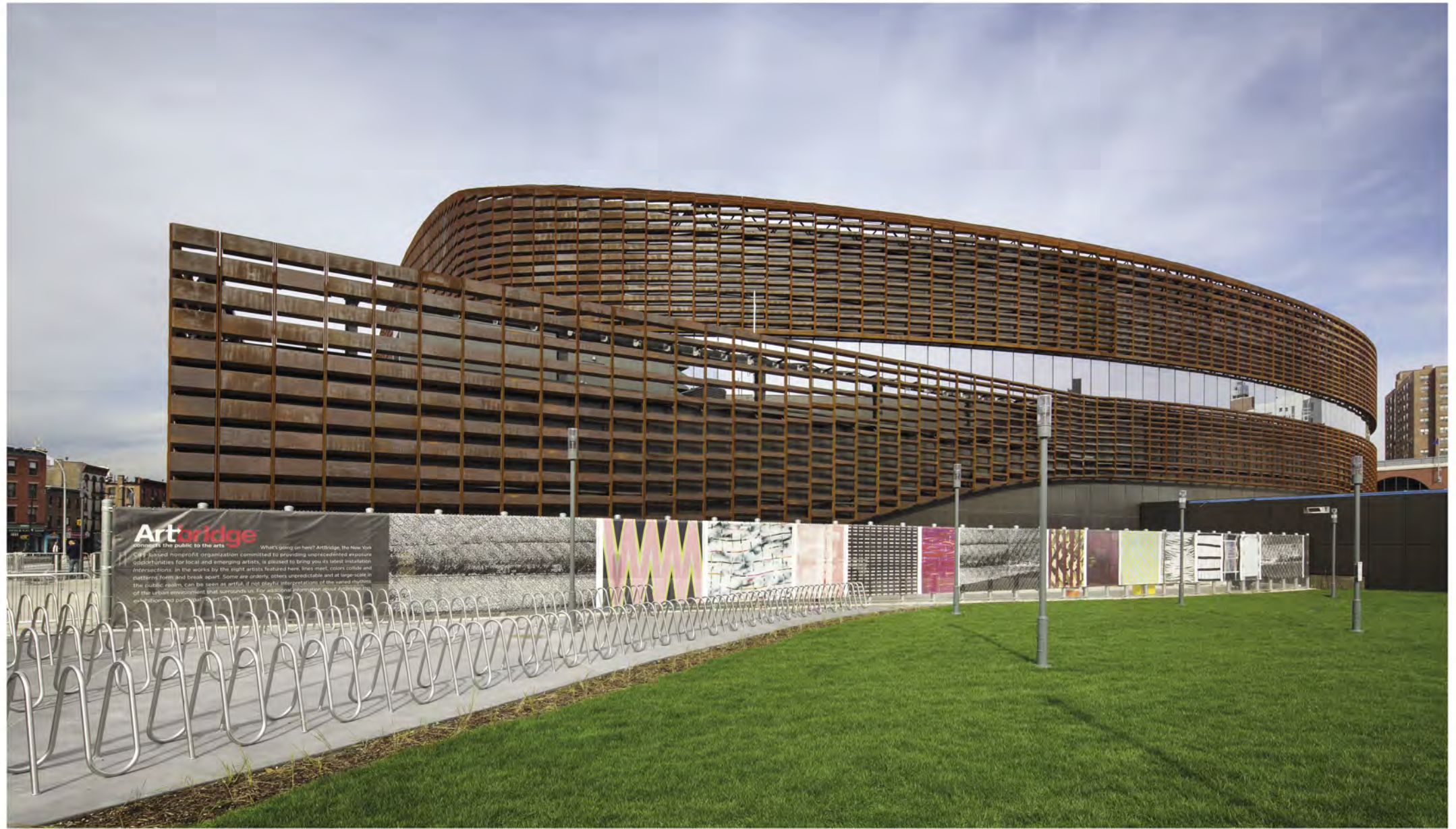
Above Internal truck elevators and turntables eliminated the need for ramps to loading docks, allowing the arena to have more of a storefront presence in downtown Brooklyn.
