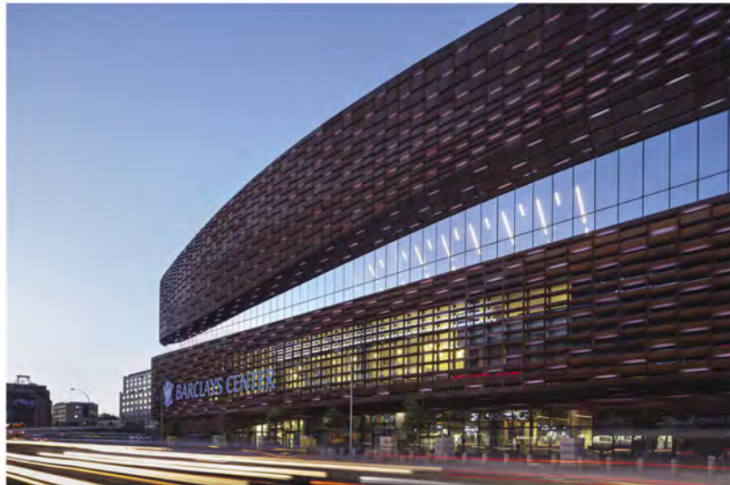
Above Panels cover 85 percent of the arena's facade. The steel shroud helps to break down the scale of the 675-square-foot building.
