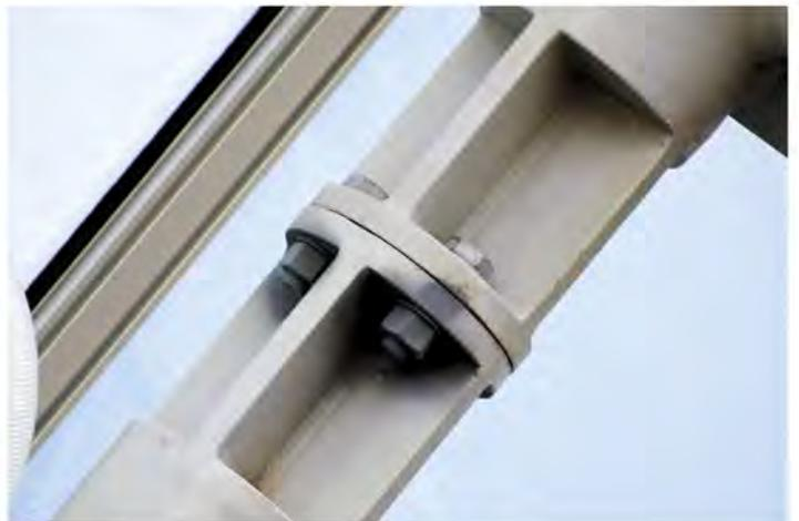
**Above** A system of 8-inch-diameter steel arches and 4-inch-diameter purlins created efficient geometric connections, reducing construction costs.
