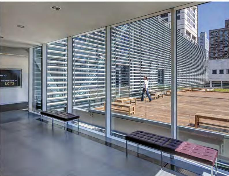
This page and facing top A brise-soleil of square aluminum bars shields the theater's north, east, and south sides, contributing to its LEED Silver rating and helping it blend with the Saarinen-designed structure below.
