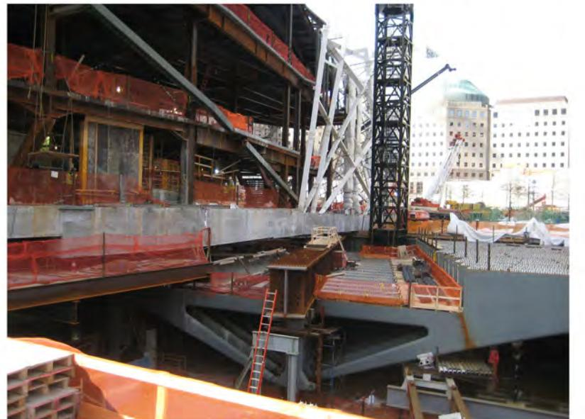
lateral loads to the PATH girders and onto the plaza structure at the south side. Standing adjacent to the newly reconnected Greenwich Street, the east facade conforms to the site-wide security requirements.
