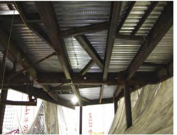
This page, clockwise from top A mechanical opening in the transfer girder. The memorial's northeast plaza and mechanical plant. Structural support for the mechanical floor.
