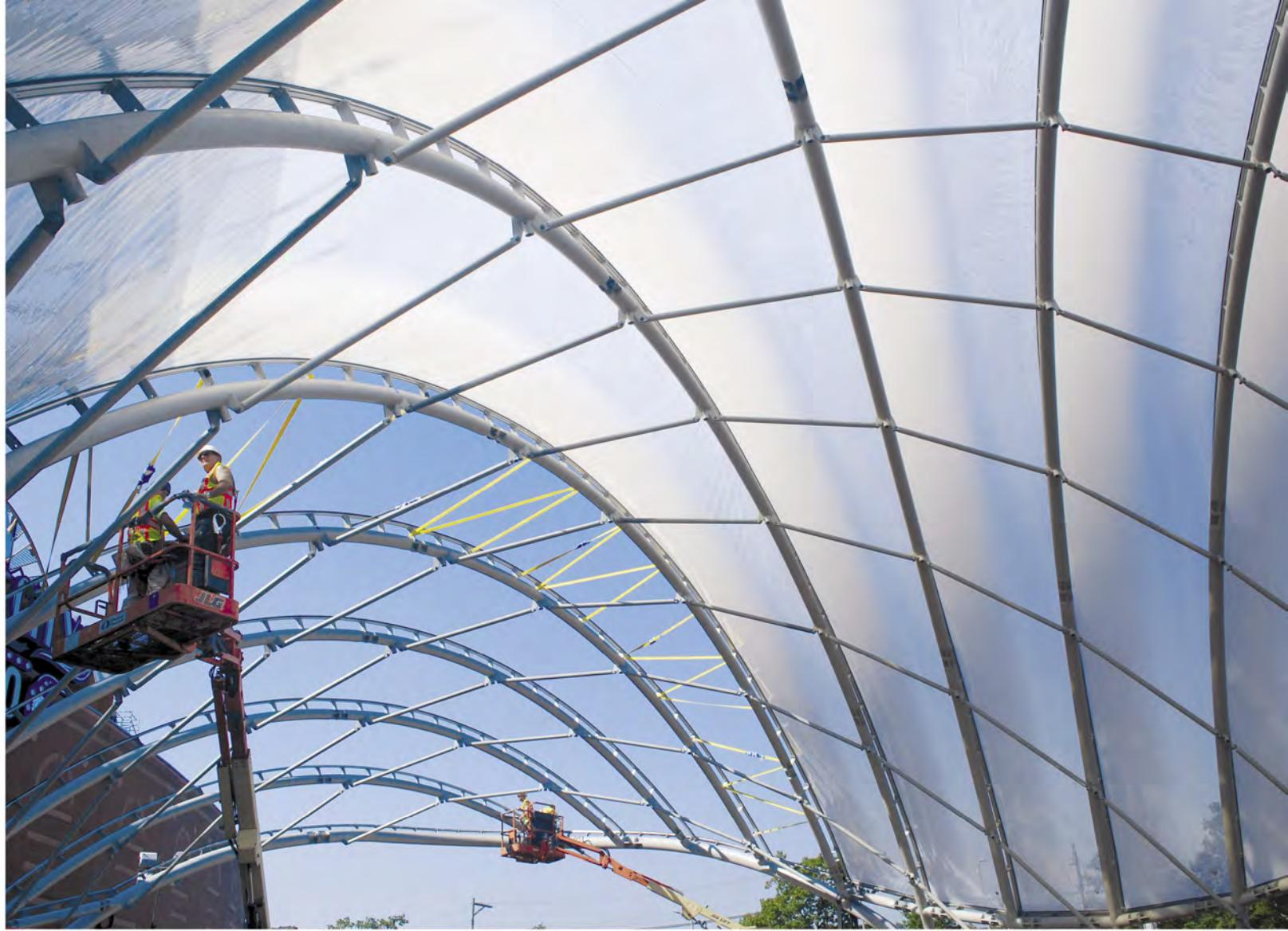
**This spread** The 11,000-square-foot porte-cochère is a steel lattice shell structure covered with ETFE, a transparent film that is lightweight, flexible, and sustainable. Installers feed the edge of the ETFE film into the clamp bar of a 6-inch steel extrusion designed to hold the material in place.
