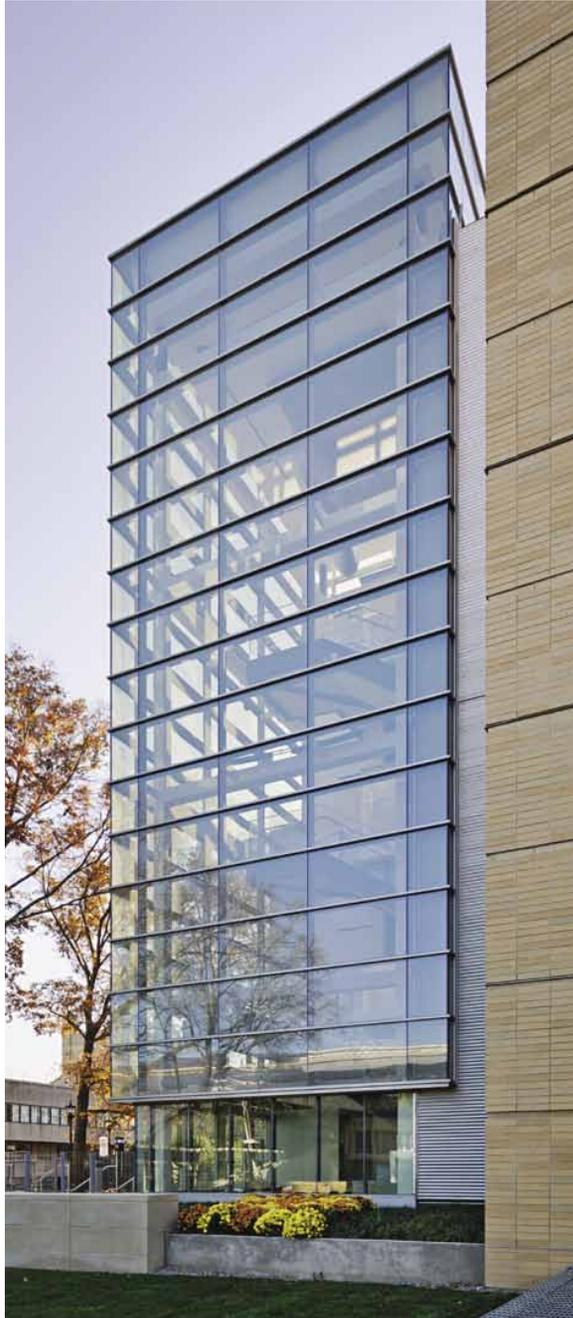
**Left and facing** The curtain wall is a stick built, field glazed system with mostly vertical mullions spanning at least two floors, supported at the edge of slabs. Vented shadow boxes were part of the spandrel conditions of the curtain wall. Extensive decorative metal was used at the exposed areas of the curtain wall, to accentuate its distinction from the masonry plane.
