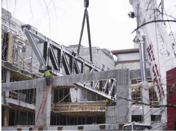
**Left** At the fourth floor, three 10-to-12-foot deep transfer trusses were installed to make the clear-span space for an 800-seat auditorium.
