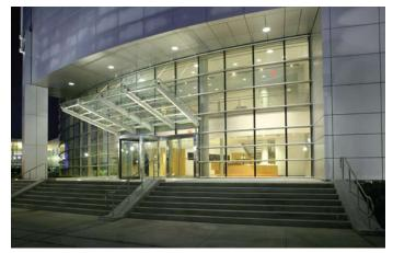
Above The entry canopy is supported by custom tapered structural steel; 2½inch steel pipe runs perpendicularly through the members. The frame is sus-pended by %-inch-diameter stainless
