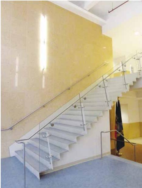
**Left** The stair's top riser and tread are welded to a lateral beam with its flange removed. The construction allows the stair to function as the beam's top chord, creating a less bulky design.
