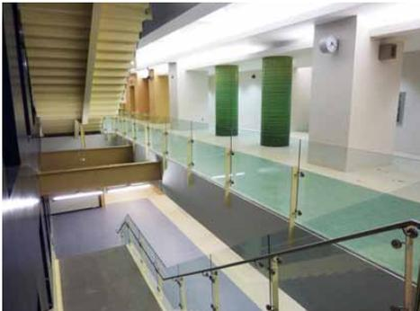
remaining column adjacent to the stair opening was supported laterally by steel beams at each level, so Ciardullo, also the project's structural engineer, had to calculate how many beams could be removed to create the opening.
