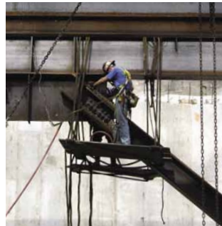
Left The curtain wall's vision panels have a low-e coating and 43 percent visible light transmittance. Above Steel erectors construct outrigger trusses at the sixth floor.
