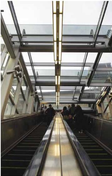
and the glass roof panels have an additional 60 percent frit pattern added to that, computational fluid dynamics studies showed that without some openings the interior would be unacceptably hot in the summer. Each of the domers has a 1-foot high opening along three sides to allow heat to escape. The panes of roof-glass cantilever over the openings, and offer some protection from the weather.
