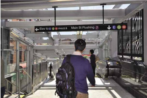
**Left** The designers devised a roof made up of a series of glass domers to allow greater headroom over the escalators. The space just beneath the purlins is open to allow this volume to be naturally ventilated; the fitted glass is cantilevered over this space to protect it from the weather.
