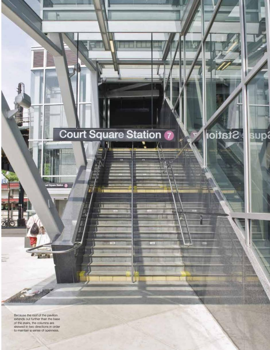
Because the roof of the pavilion extends out further than the base of the stairs, the columns are skewed in two directions in order to maintain a sense of openness.
