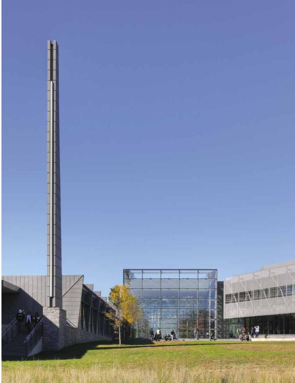
Left A 60-foot-tall tower framed in steel and clad with zinc panels anchors the facility's south wing.
