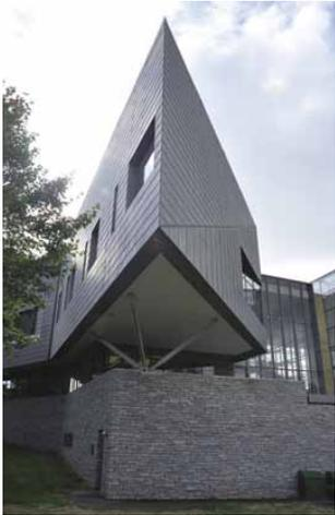
a ladder in construction. Each leg terminates in a steel pin detail that eliminates bending forces in the tripod. A plate assembly at the base ties the 4-inch-diameter pins together, transmitting gravity and lateral forces to the foundation.
