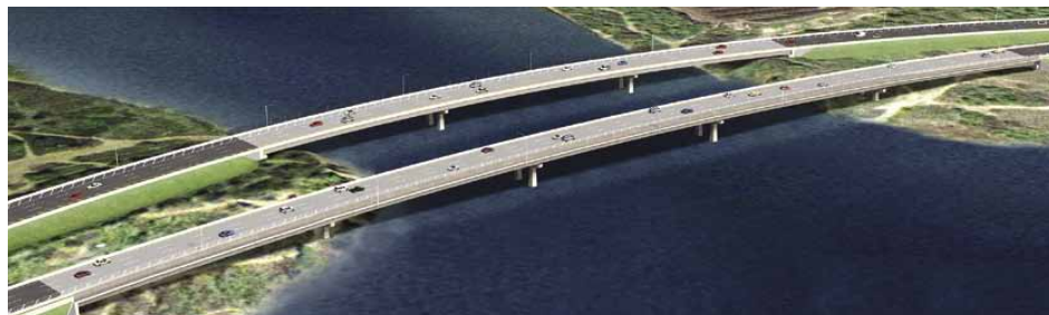
Above The existing Paerdegat bridge (top) and renderings of the new east- and westbound crossings, scheduled for completion in the summer of 2012.
