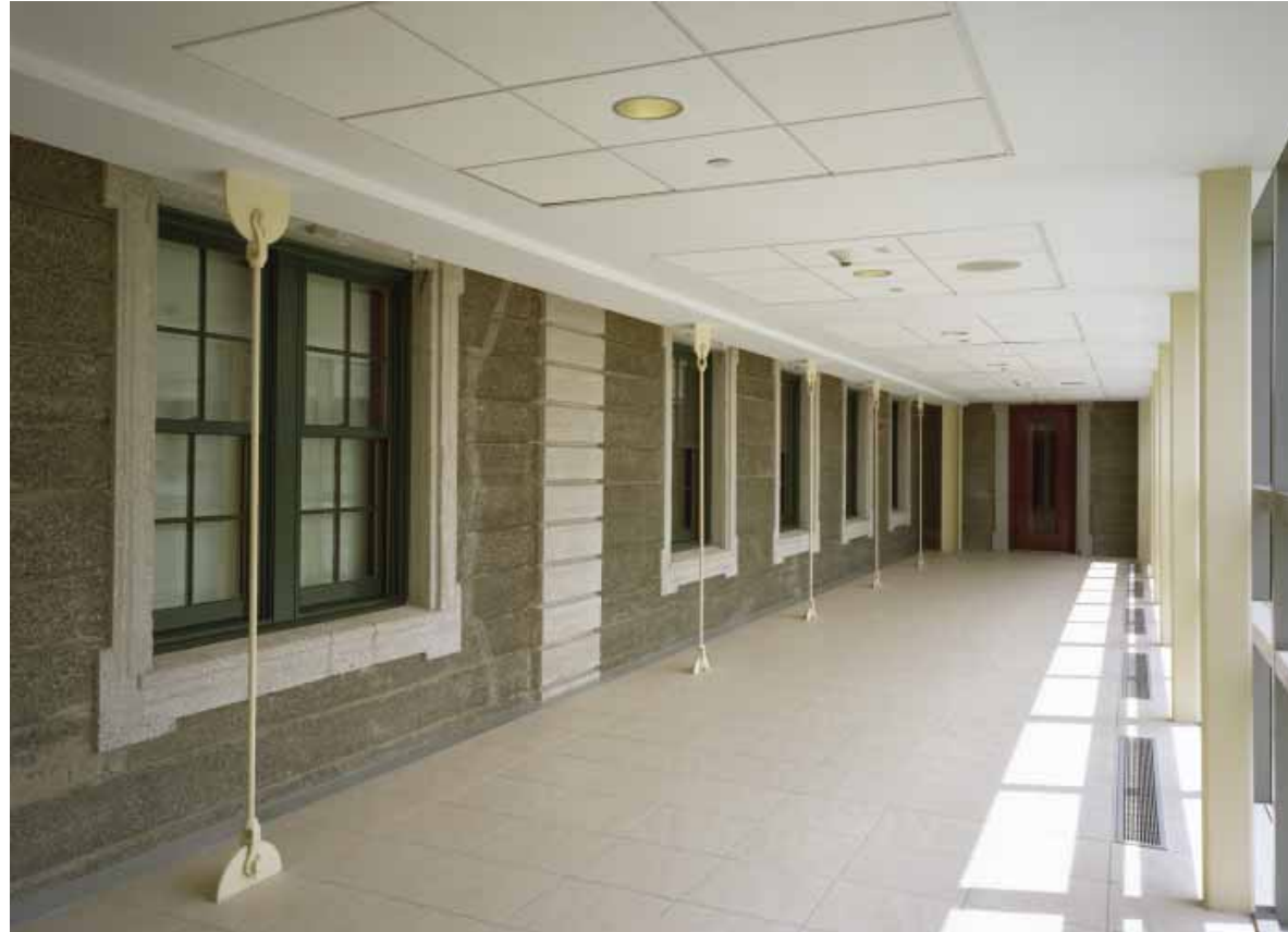
Above The annex and connective corridors were constructed while the decaying original structure was reinforced.
