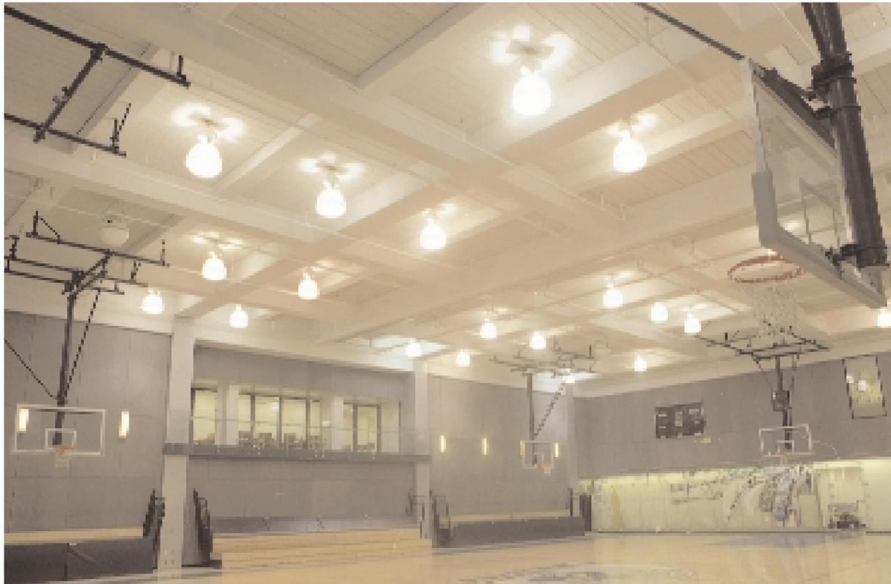
Over the gymnasium, four steel trusses provide an 85-foot clear span for the space while supporting a 4,200-sq.ft.elevated courtyard.
