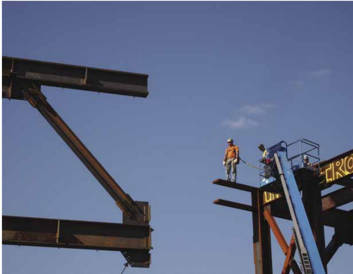
**This spread** Massive steel trusses allow the building's 95-foot cantilever, which creates a protective overhang above the main entrance and maximizes the long, narrow site.
