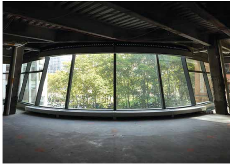
Clockwise from top left In the cones, the spandrels are frosted panes of glass illuminated by interior LED covers. Sections of the podium cone (left) and of the tower cone (right). The cones create uniquely curved window bays at each floor. The building's structural system consists of a concrete core with steel framing.
