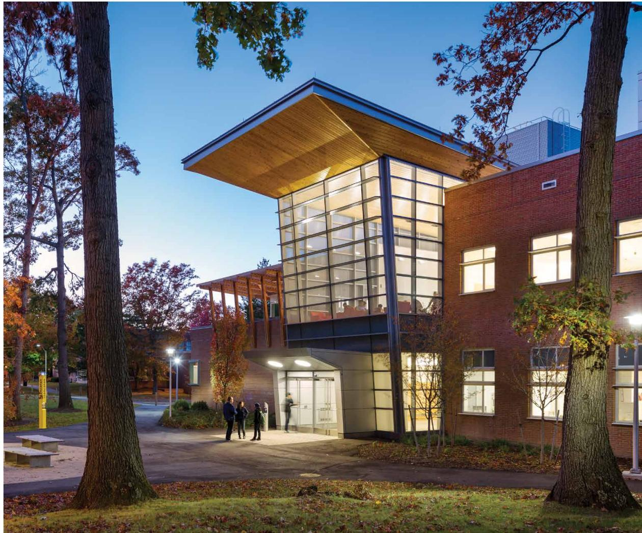
A pair of tapered W21s clad in cedar cantilevers 20 feet beyond the south elevation of the New Computer Science Building to provide a public entrance canopy.
