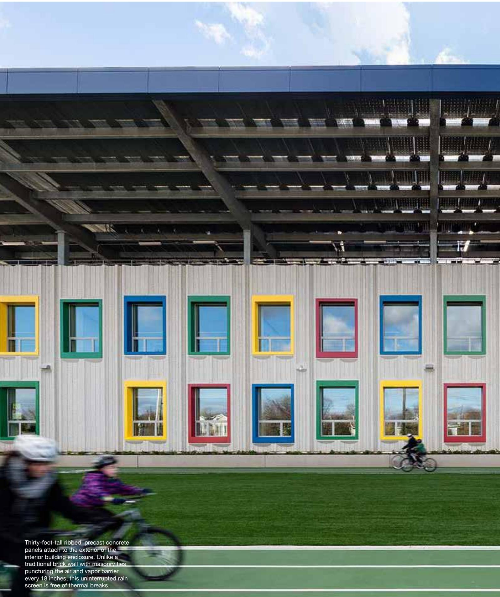
Thirty-foot-tall ribbed, precast concrete panels attach to the exterior of the interior building enclosure. Unlike a traditional brick wall with masonry ties puncturing the air and vapor barrier every 18 inches, this uninterrupted rain screen is free of thermal breaks.
