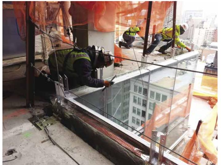
**Clockwise from top left** Exterior façade inspections of the glass and joints. W&W Glass's team sets the unitized panels from a mobile mini-crane with winch positioned three floors above. The installers seal the tops of the unitized panels in preparation for the next floor of panels to be set. Panels are erected by a mini-crawler crane at the building podium.
