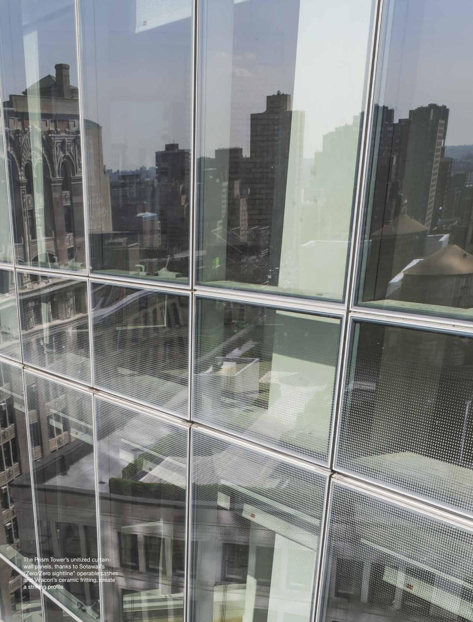
The Prism Tower's unitized curtain-wall panels, thanks to Sotawal's "Zero/Zero sightline" operable sashes and Viracon's ceramic fritting, create a striking profile.
