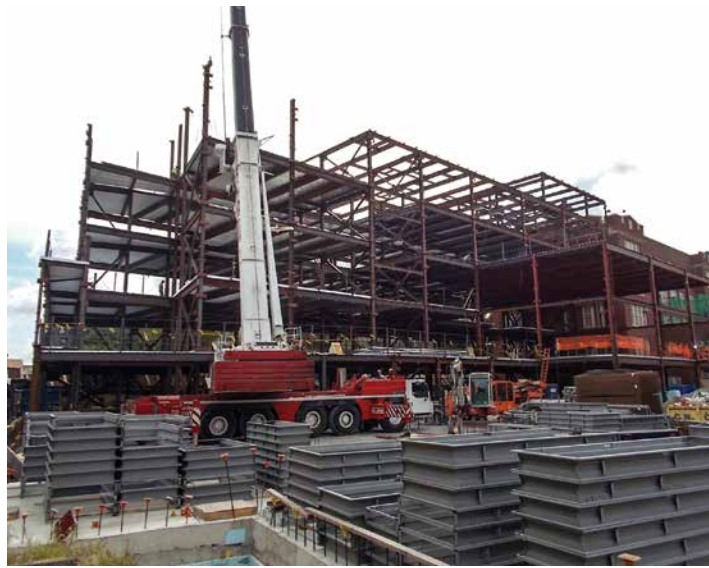
An adjacent train line made erecting the steel structure a challenge, requiring flagmen provided by MTA and specialized staging.
