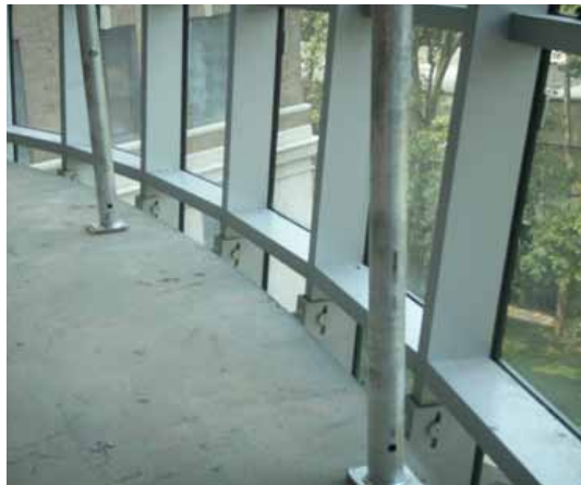
Above A section detail of the west curtain wall's curved portion. Below The structurally exposed slotted stainless steel connection allowed bolts to be tightened as the structure settled, ensuring a watertight facade.
