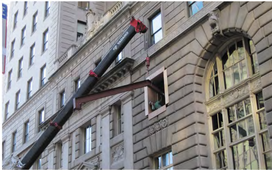
Left Steel framing for the gymnasium roof is lifted through the third-story windows of 26 Broadway and carried through the building into the courtyard. Below Five W18x86 wide-flange beams are welded to the building's original steel columns to create the roof of the gymnasium.
