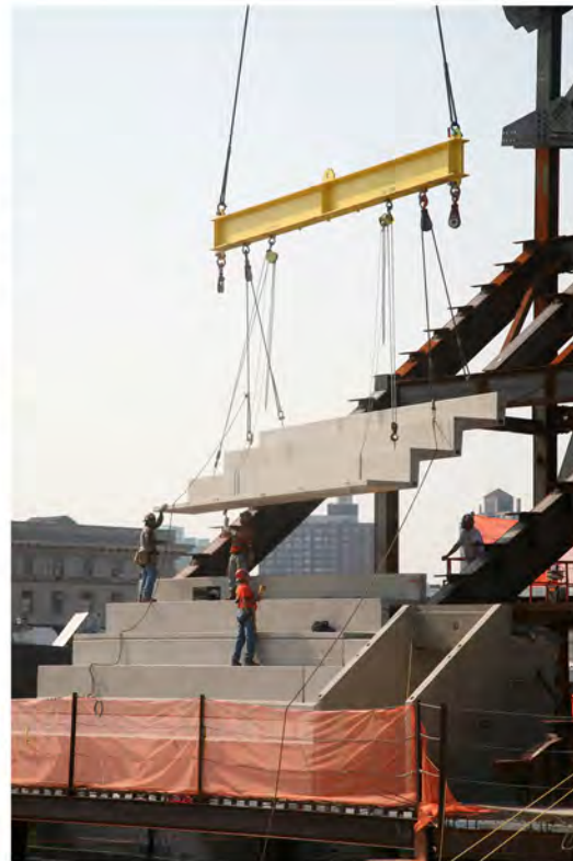
Above and left Precast concrete stadia units span between steel rakers. Far left The steel erection sequence minimized strain compatibility between elongation of the roof structure's tension tie and the superstructure's lateral displacement.
