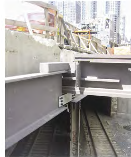
This page Steel box girders and precast concrete panels support the first five floors over an Amtrak tunnel.
