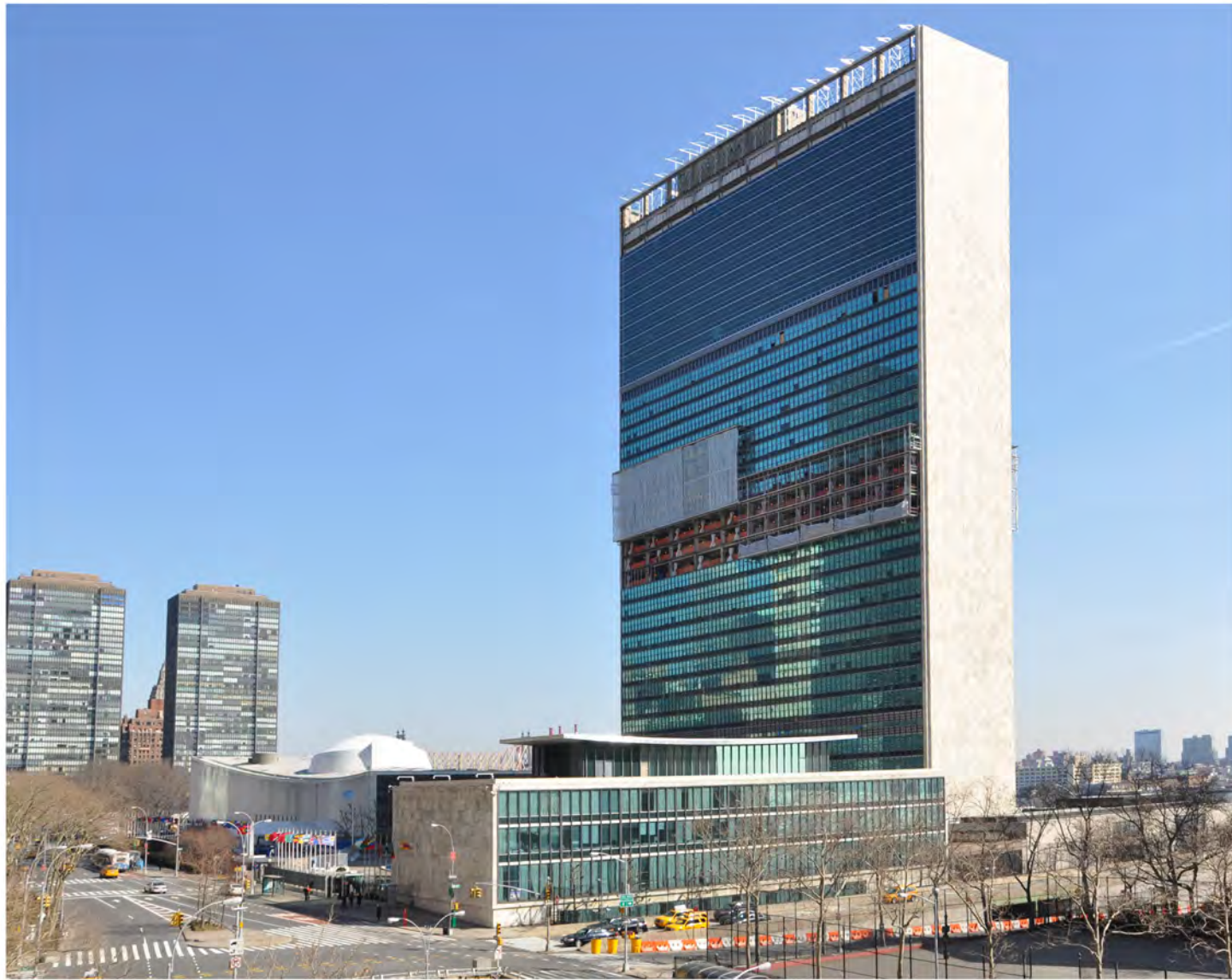
Above Completed in 1952, the Secretariat was the first skyscraper in the world with a curtain-wall enclosure. Left The recladding is part of a $1.87 billion renovation of the UN's New York City compound.
