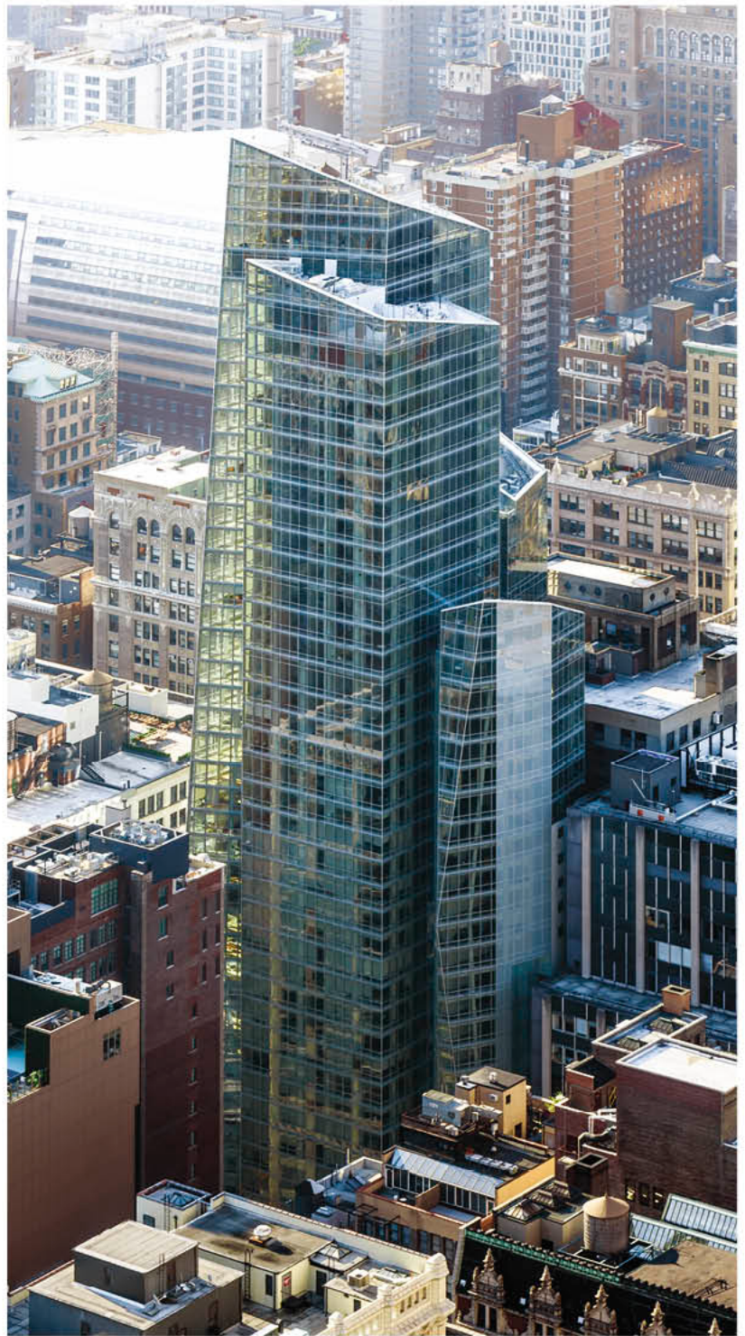
Above Christian de Portzamparc's design, assembling the building out of four main volumes and optimizing internal light penetration, means that nearly every floorplan is unique and calls for extensive customization of curtain-wall components.
