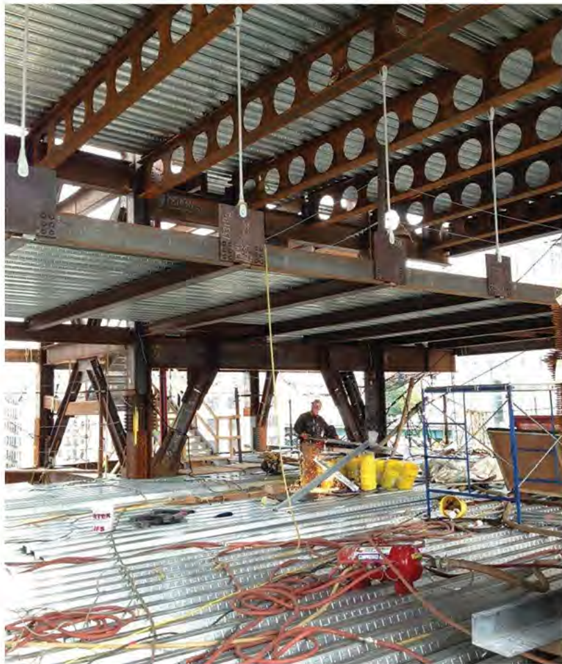
Clockwise from top right A model of Lenfest's structural steel framing. Large cellular beams running north-south retain strength with less mass and allow ducts, piping, and conduits to pass through the round openings. Lenfest under construction, looking northeast. Facing from top The Katharina Otto-Bernstein Screening Room. A north-south section depicting Lenfest's varied programming.
