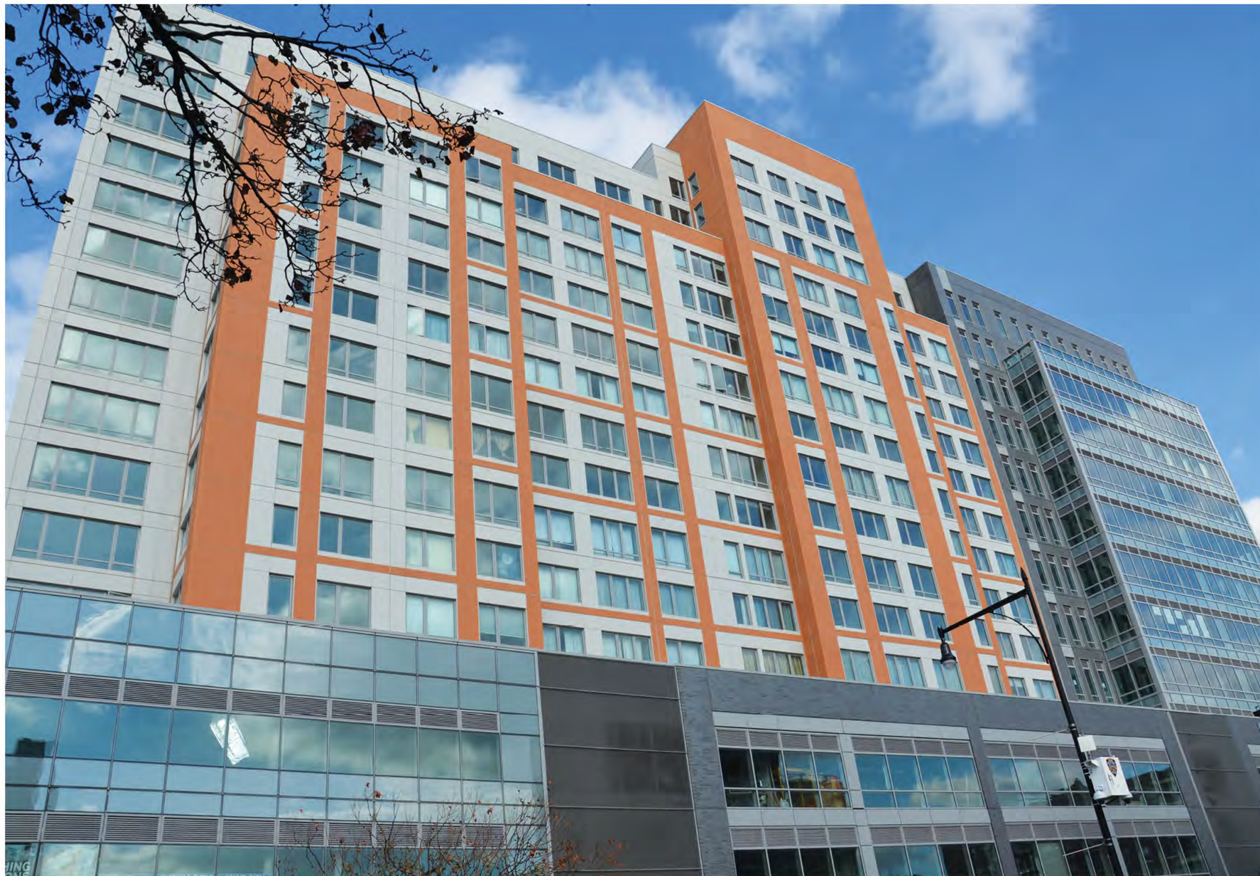
A residential tower and commercial building are the first phase of the 1.8-million-square-foot Flushing Commons mixed-use complex at Union St. and 39 th Ave.
