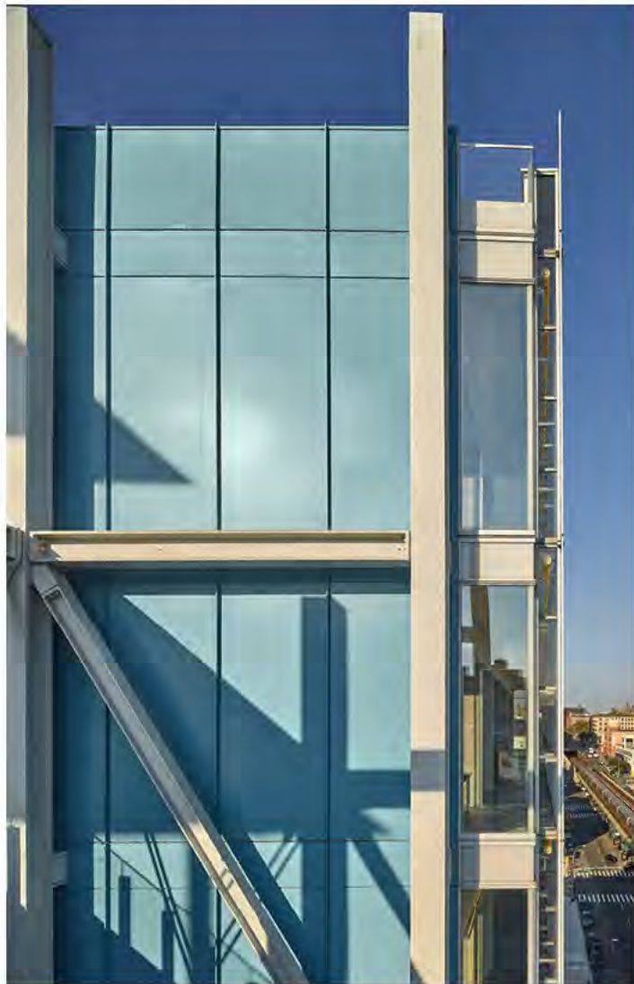
Top Vibration support for Greene's cooling towers. Above Several facade typologies help optimize thermal, environmental, and acoustic performance.
